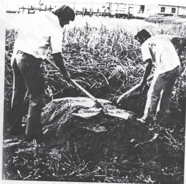
Smoothing top of first rock to allow for more height.
